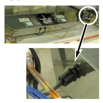
**Lift fan plenum up and back to remove.** (view is from the back)
